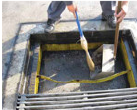
Figure 5-19 Storm drain screens to accumulate plastic pellets.
