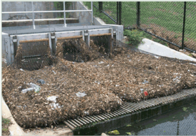
Figure 6.4-3. Picture of end-of-pipe trash net containing trash.
