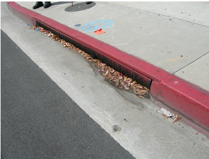
Figure 6.4-2. A catch basin brush insert with accumulated debris
